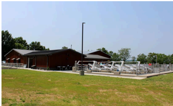
Figure 9 Leitchfield Water Treatment Plant
