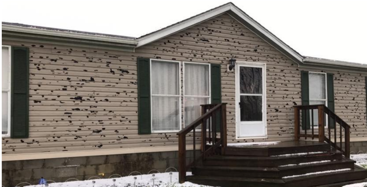
Damage to a residential structure after an April 2017 Hailstorm in Nelson County. Source: WLKY
